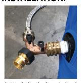
1. Attach the nipple, swivel and Y valve to the input side of your system as shown (left when facing) and familiarize yourself with lever operation.
